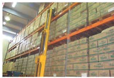
State of the art warehousing infrastructure
